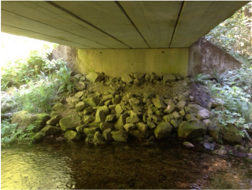
Left Bank Abutment when facing downstream
