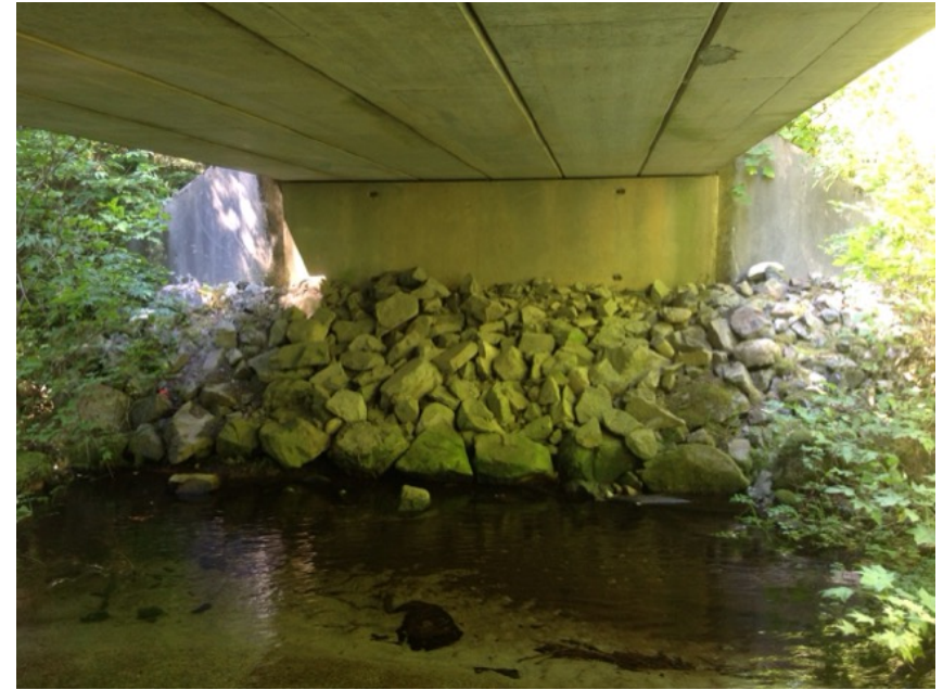
Right Bank Abutment when facing downstream
